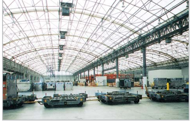
United Airlines Cargo Facility at JFK Airport in New York, USA.
