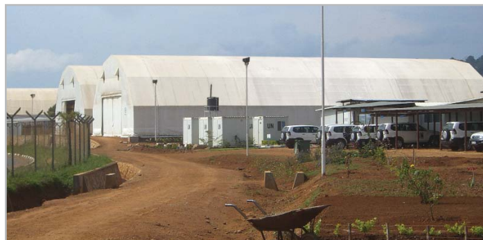
NV buildings, Entebbe, Uganda. 20m wide x 42m long with 4m side wall. Used for the UN mission in Congo (MONUC).
