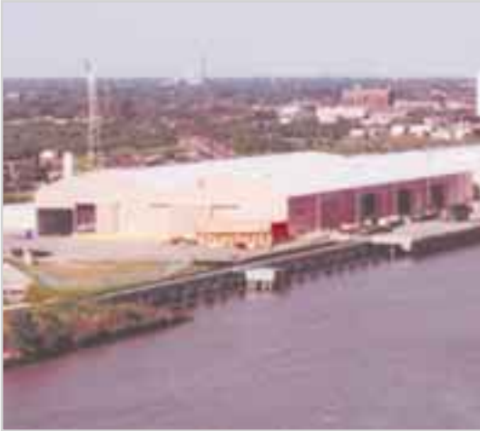
Right: Port Arthur, USA A 220' (67m) x 525' (160m) BVE Twin-link building provides an additional 115,500 ft 2 (10,720 m 2 ) of transit storage in addition to covering the port's railroad siding.
