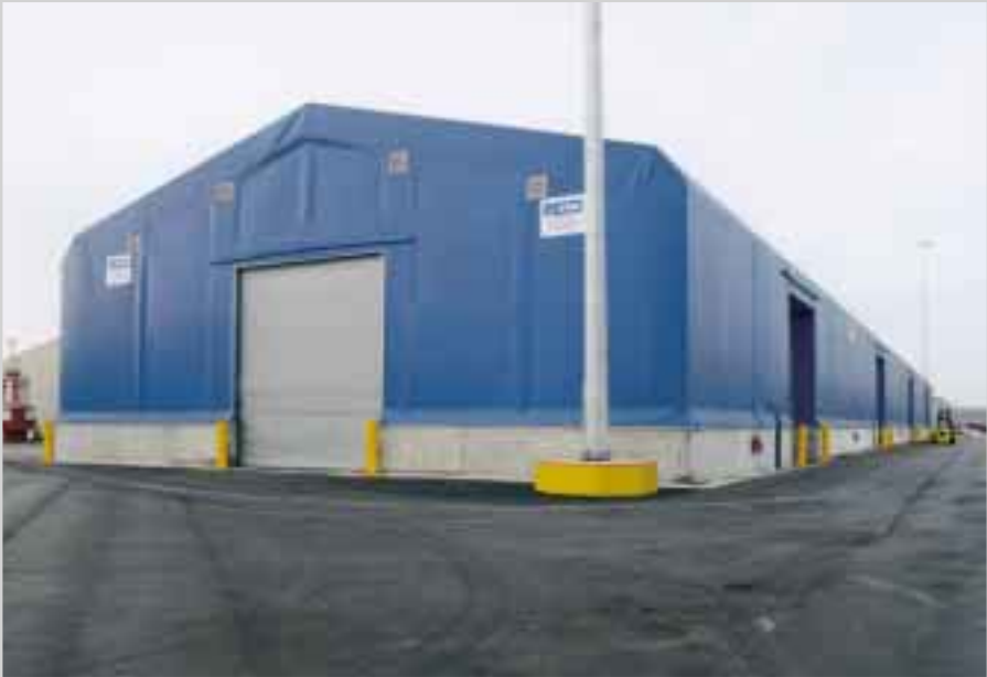
Above: Belfast, Ireland, UK. Measuring 78' (24m) wide x 148' (45m) long, with 20' (6m) sidewalls, this building was delivered and erected within eight weeks from receipt of order, and included lighting and ventilation.
