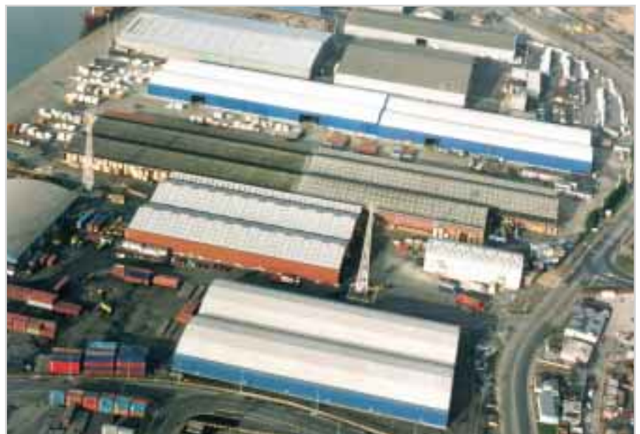
Left: Londonderry, UK. A substantial warehouse measuring 131' (40m) x 475' (145m). To maximize internal storage space the building is constructed with I-Beam column walls as an alternative to the traditional 'lattice' design. Reason for choosing Rubb - versatility.
