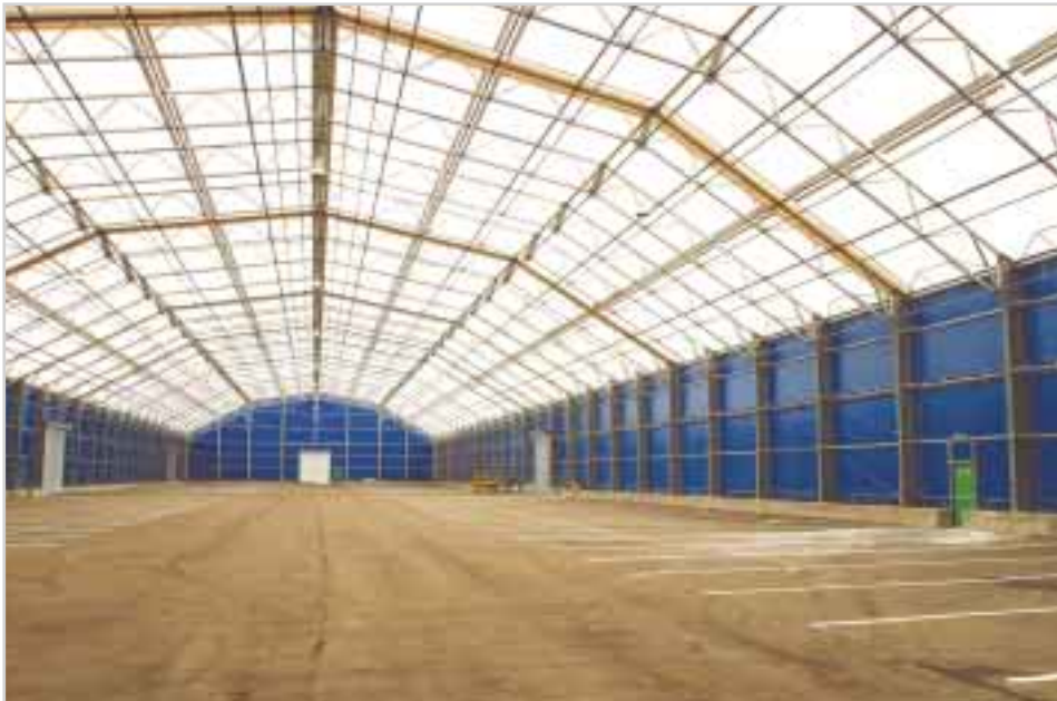
Left: Londonderry, UK. A substantial warehouse measuring 131' (40m) x 475' (145m). To maximize internal storage space the building is constructed with I-Beam column walls as an alternative to the traditional 'lattice' design. Reason for choosing Rubb - versatility.
