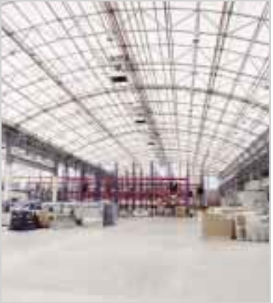
Right: Virginia International Terminal, Norfolk Virginia, USA. 156,000 ft 2 (14,500 m 2 ). Rubb buildings can be linked together to create virtually any amount of open storage space as the photo below shows
