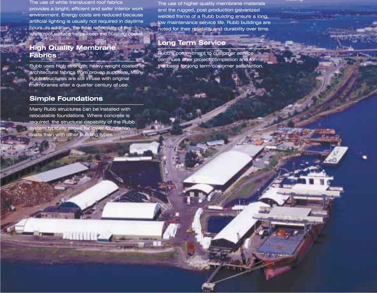
The first building at this site was erected in 1984 and is still in use today with original membrane cladding.
