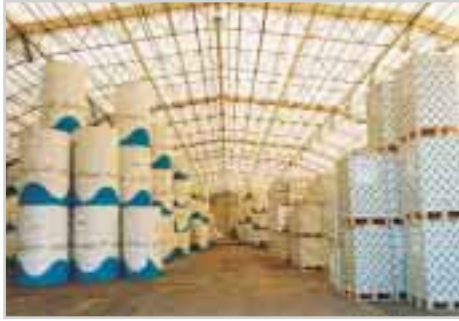
Above: Convoys, Chatham Dock, UK. This 115' (35m) x 360' (110m) BVE building shows how bright a Rubb building can be without the use of artificial lighting.
