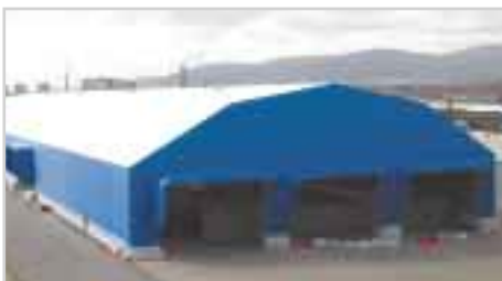
Above: Belfast, Ireland, UK. This warehouse measures 148' (45m) x 575' (175m). Like Londonderry it is constructed with column walls and has 6 individual 40' (12m) openings with canopies for ease of access.
